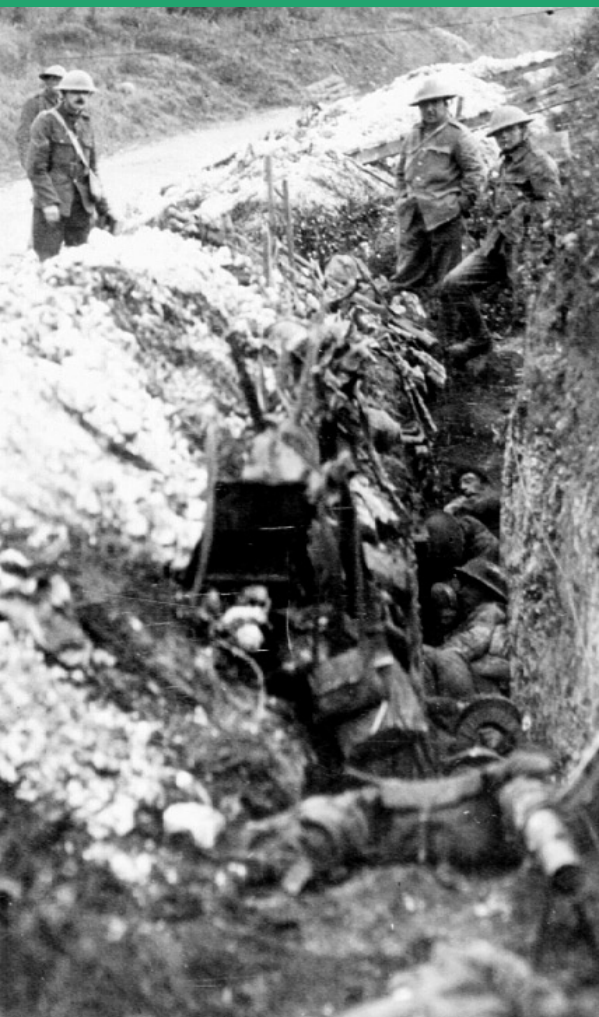
St. John's Road Trench, 1916
