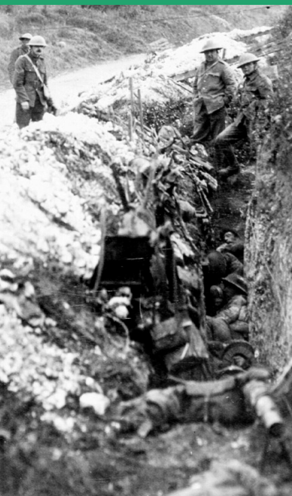
Tranchée St. John's Road, 1916
