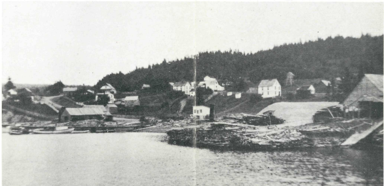
The village of Charlottetown on Clode Sound near the National Park
