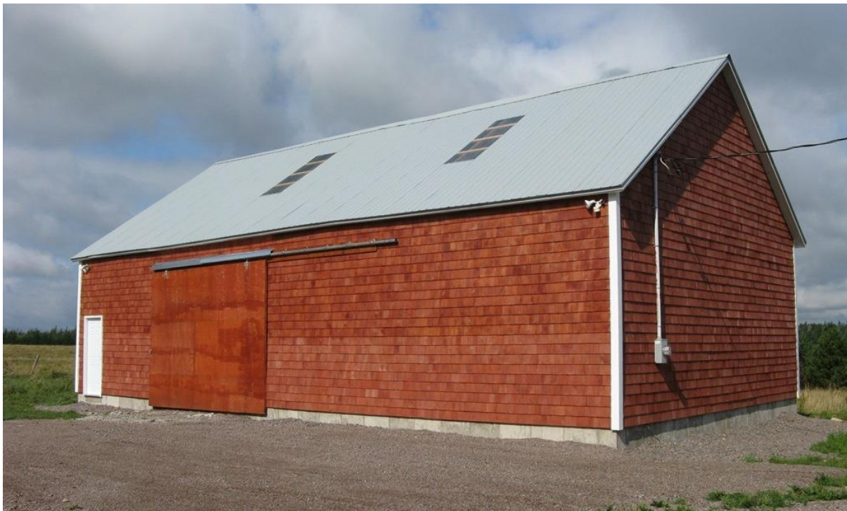
Figure 9: Storage barn, 607 Luciphy Road, Tintamarre NWA
