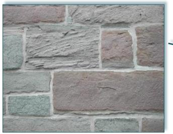
Figure 8. Stone blocks made of Sillery sandstone (Photo by Léopold Nadeau, Geological Survey of Canada, 2006)
