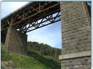
**Figure 50. Granite blocks forming the pillars of the Quebec Bridge** (Photo by Léopold Nadeau, Geological Survey of Canada, 2007)
