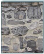
Figure 13. Blocks of black argillaceous limestone, "Black Cap stone" (Photo by Léopold Nadeau, Geological Survey of Canada, 2006)
