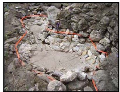
Pond Rehabilitation work, 2004
