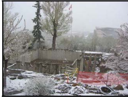
Foundation for reconstructed Cottage at Reader Rock Garden, 2004
