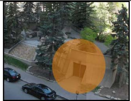
Door to Parks Office at Century Gardens, 2007
