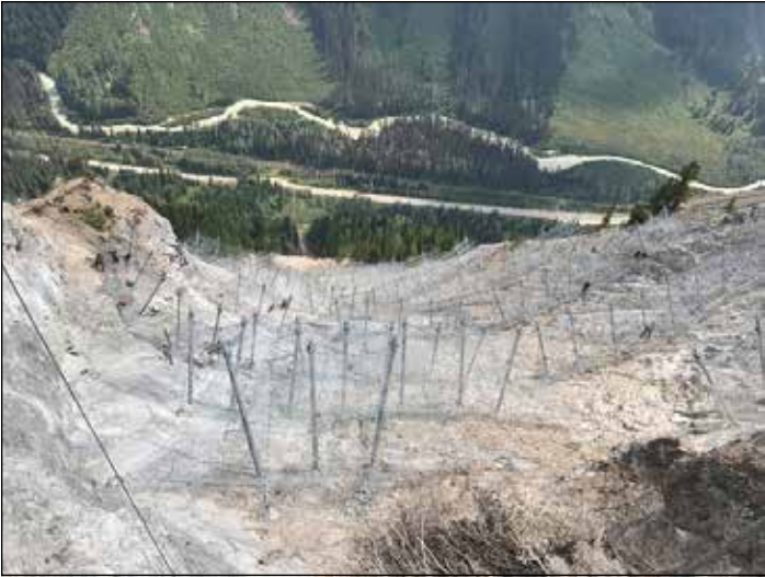
Figure 3: Installation of snow nets in Cougar Corner, 10 km west of Rogers Pass (source: Brian Gould, Alpine Solutions Avalanche Services)
