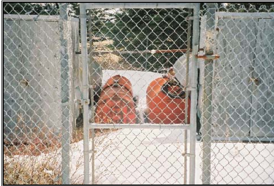
Photo 3. Aboveground storage tank and fuelling facilities
