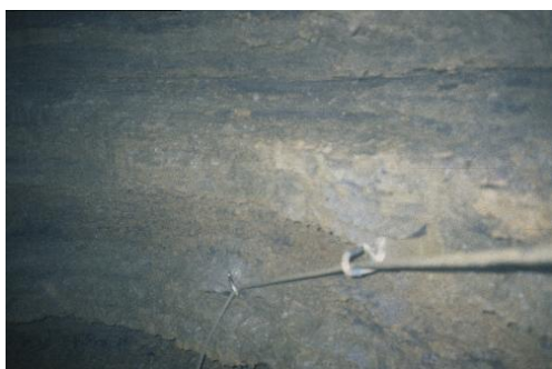
Figure 135: There is solid rock somewhere underneath. Not far between bolts here! (Marek: CC05-04-0079)
