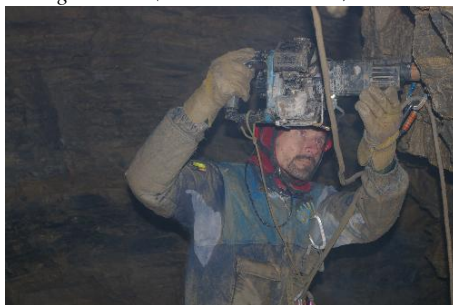
Figure 146: Setting the permanent bolts. This has to be just right... (Christian: CC05-107)
