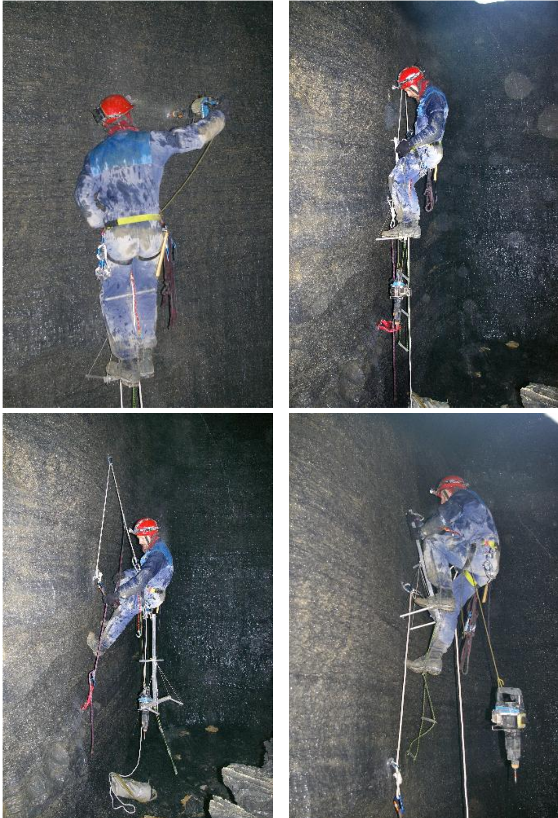
Figure 20: Marek on the bolting platform, showing the sequence (clockwise from top left): Stand on platform; drill hole; hang from safety rope while dismantling platform and climbing up; climb onto platform using its short etrier. After that—next hole! (Christian: CC05-058, 059, 060, 061)
