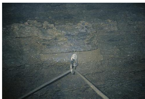
Figure 136: Spot the missing block—the bolt is now on what was behind the loose rock, and the original hole is visible above it (Marek: CC05-04-0081)
