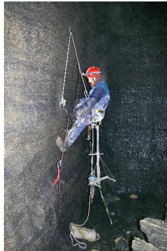
Figure 102: Platform loose, climb up the rope to the next bolt (Christian: CC05-060)
