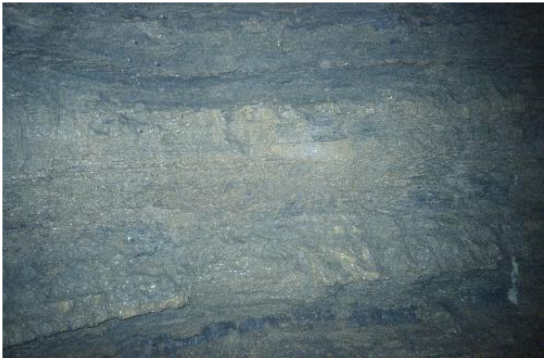
Figure 234: In the middle of this image is the place where the brick-sized rock fell out while I hammered home a bolt; the new bolt can be seen in the middle of the smooth face left behind. In the left third of the picture can be seen the drops of water on their way down towards the next climber (Marek: CC05-05-0036)
