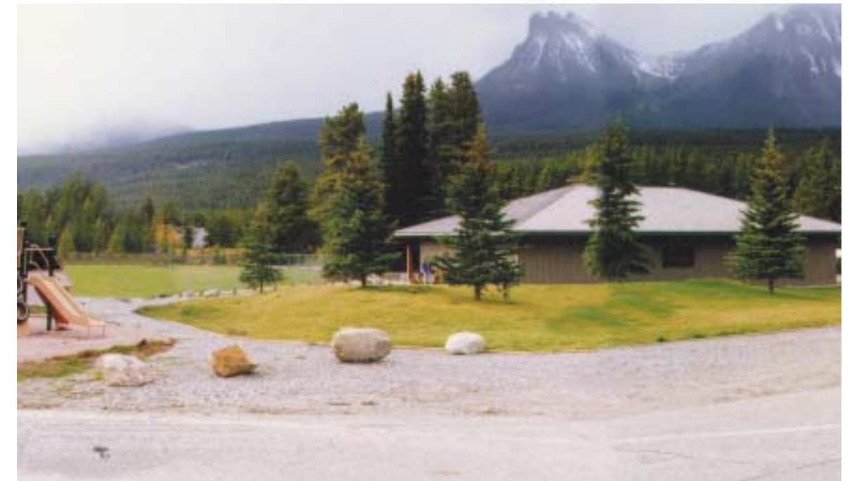
Existing Conditions - Community Centre
