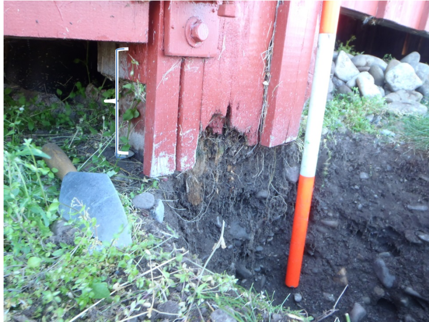
Plate 11 Southwest view of 35 cm deep test (Sub-Op U) shows pounded post as corner foundation; post is visible inside – it is rotting and not fully exposed
