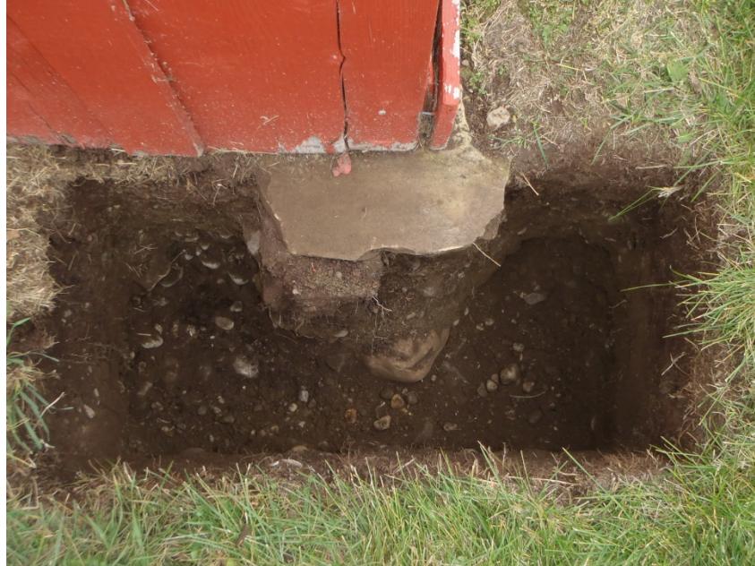
Plate 3 West view of 50 cm deep shovel tests (Sub-Ops A and B) shows sandstone foundation slab beneath corner; test is 1.0 m wide
