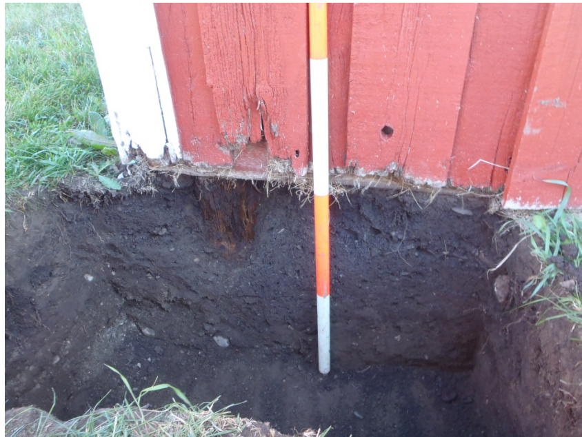
Plate 9 West view of 60 cm deep tests (Sub-Op's Q and P) shows pounded post as corner foundation; post is not fully exposed
