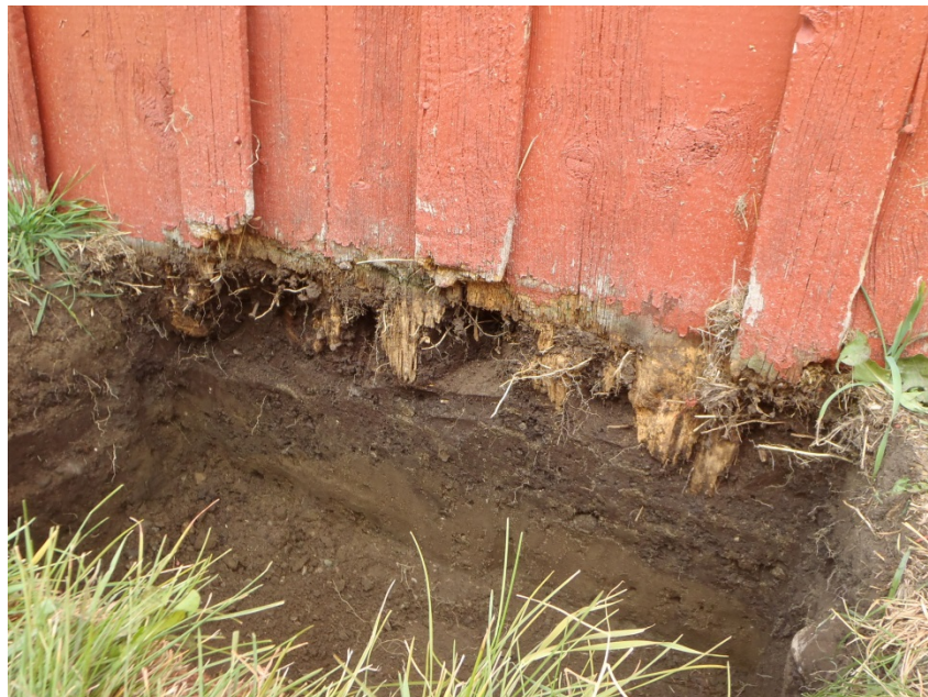
Plate 6 South view of 60 cm deep test (Sub-Op's D and E) shows rotting sill plate beneath board and batten siding; test is 1.0 m wide
