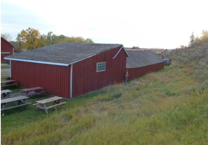
Plate 1 Northeast view of south and west façades of Historic Machine Shed; note differing rooflines indicating successive phases of building construction
