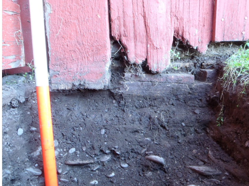
Plate 13 West view of 30 cm deep test (Sub-Op W) shows sandstone foundation slabs beneath corner; test is 1.0 m wide
