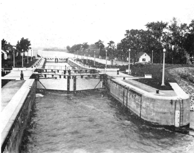
The new lock at St. Ours, 339 feet long, 45 feet wide, 12 feet deep.
