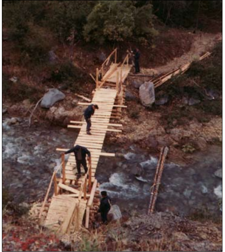
Construction of the first bridge, over Moose Creek near Lindeman, Au 1968. Yukon Corrections
