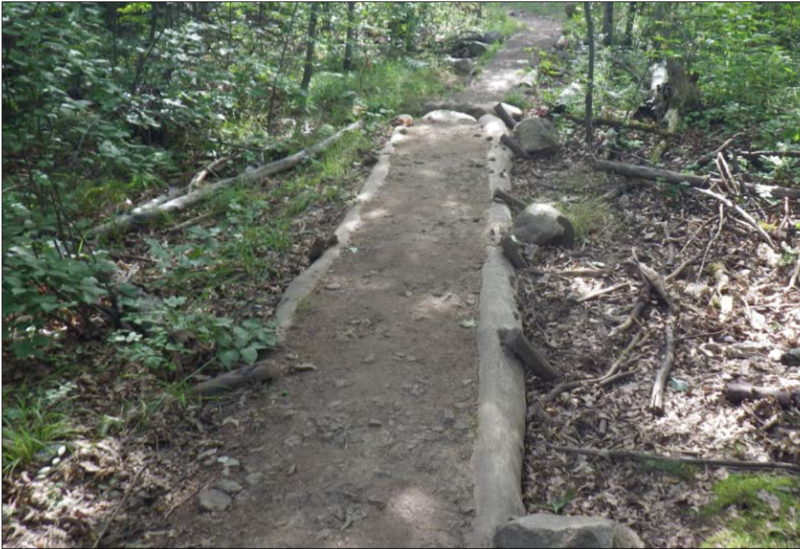
Figure 19: An example of the trail hardening undertaken by USFS portage crews on the BWCAW side of the waterway.
