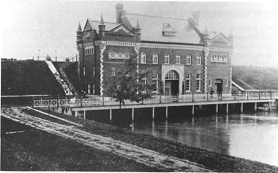
Hydro-electric power house at the Soulanges Canal in 1910.
