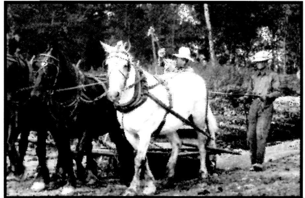
Road Construction (1930's).
