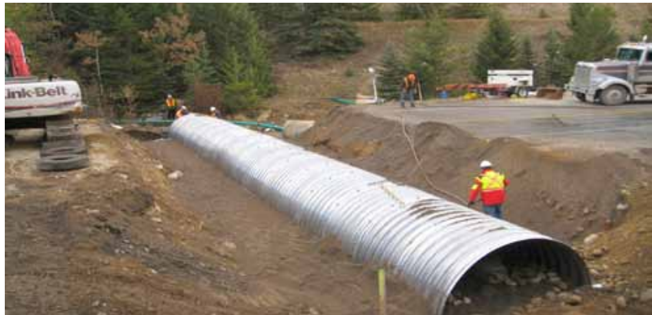
Culvert Replacement, Jasper National Park. The National BMP for Highway Infrastructure could be used to address some or all of the potential adverse effects of these types of projects.
