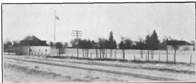
Southwest Bastion and South Wall
