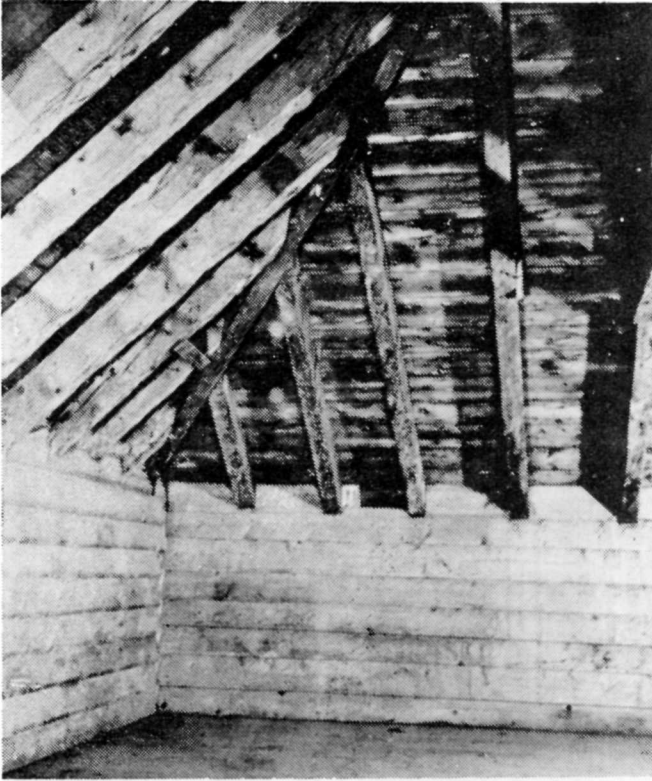
Fur Loft showing Construction
