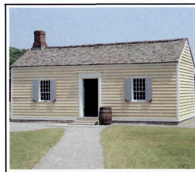
Cottages of this design were built near Fort George by local settlers or army officers desiring privacy.
