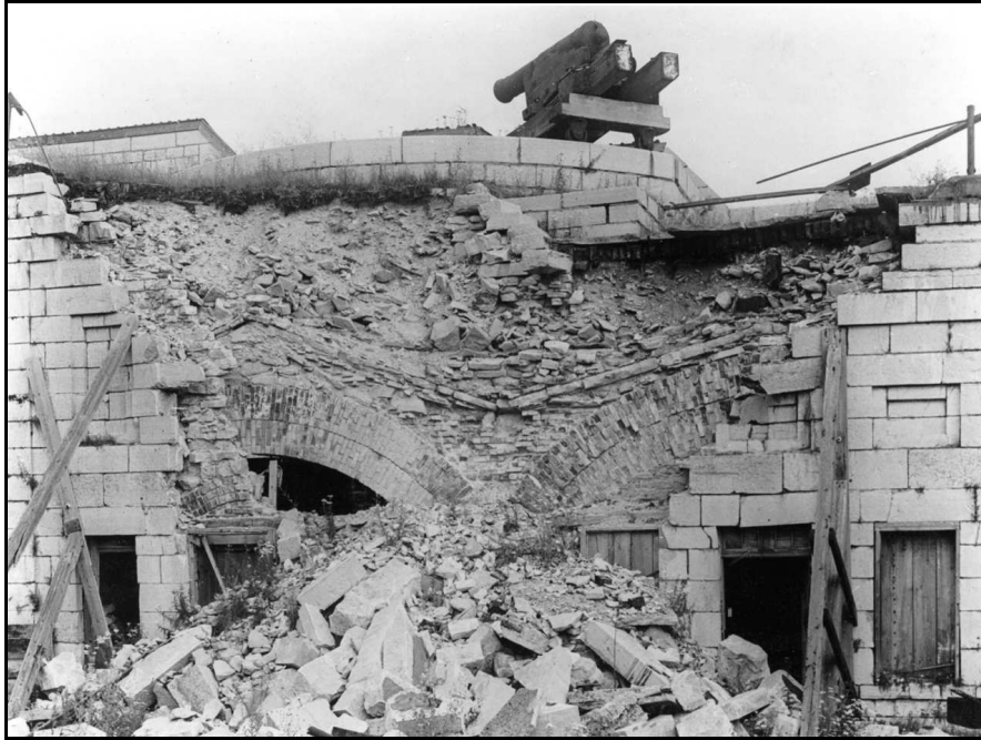
Figure 7 Collapsed section of east wall, officer's quarters. Note arches and dos d'anes, July 1931. Eric Arthur, Ontario Archives, 10002554.
