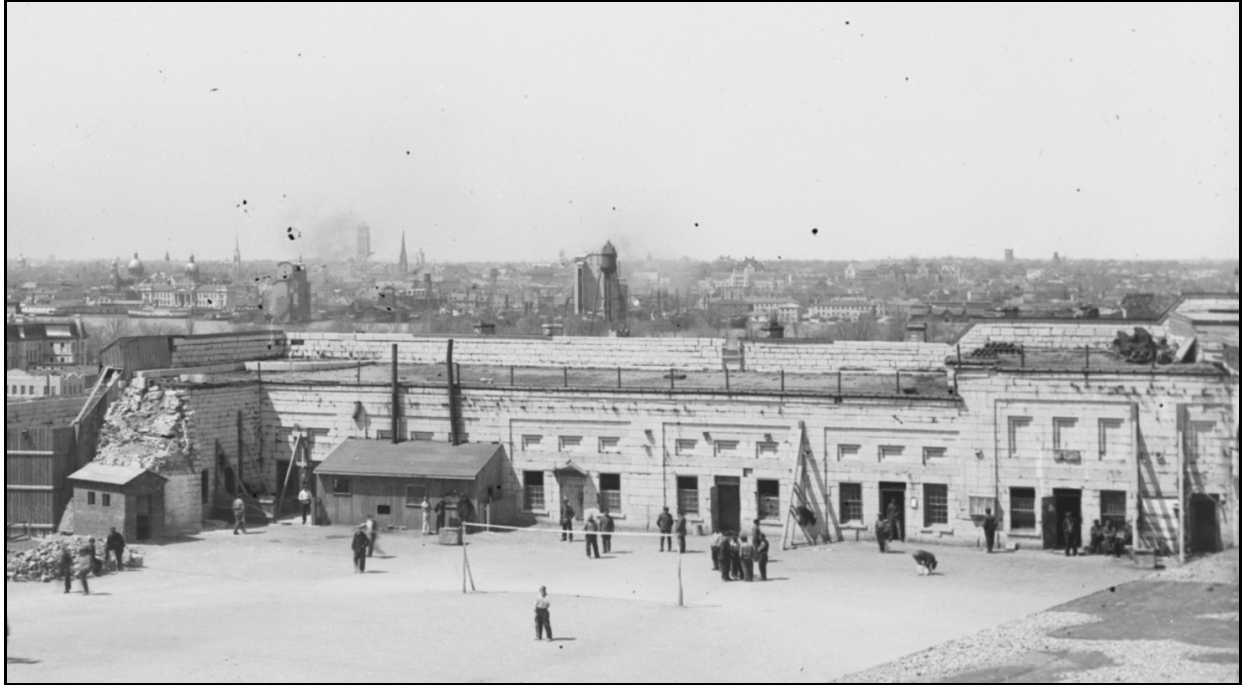
Figure 2 West wall of Fort Henry, circa 1917: note the props holding up the walls. National Archives of Canada, PA-046186.
