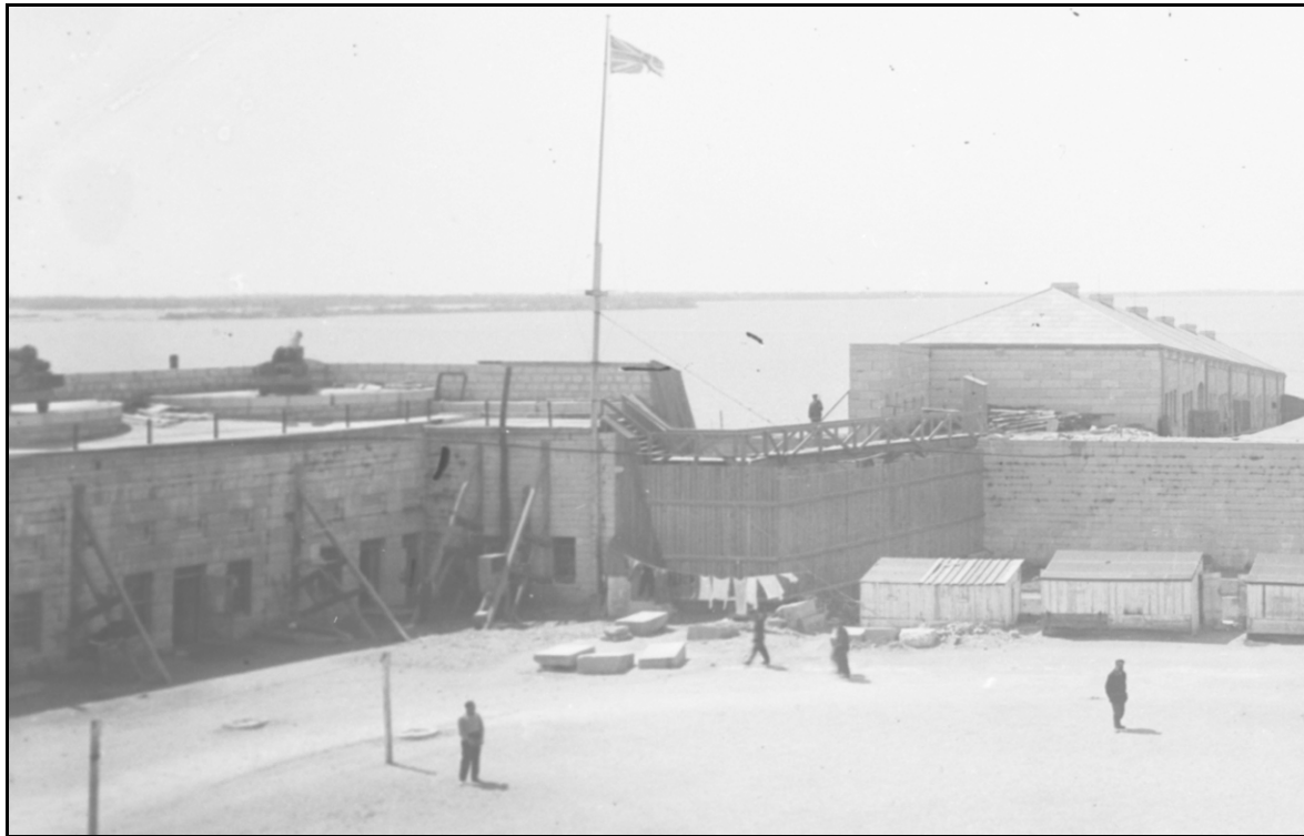
Figure 1 East wall of Redoubt, May 1917: note the props holding the wall up. Detail from G. E. Marrison, National Archives of Canada, C-043233
