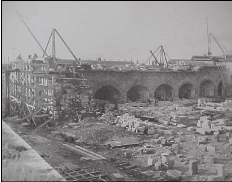
Figure 13 Officers' Quarters, west casemates, facing entirely removed. Fort Henry Archives.
