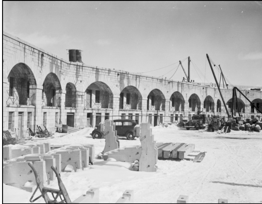
Figure 17 Interior showing north casemates, probably winter 1938. Note sheers and gun carriages. Alexandra Studio, National Archives of Canada, RD-000937.
