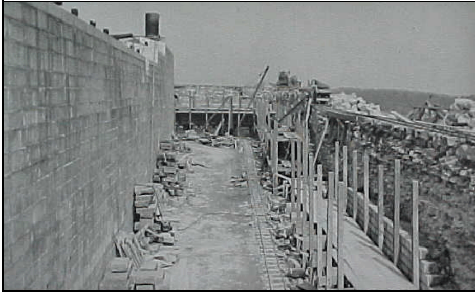
Figure 11 East ditch, looking north, reconstruction of counterscarp. Note railway to move material; facing moved forward slightly from original position. Fort Henry Archives.
