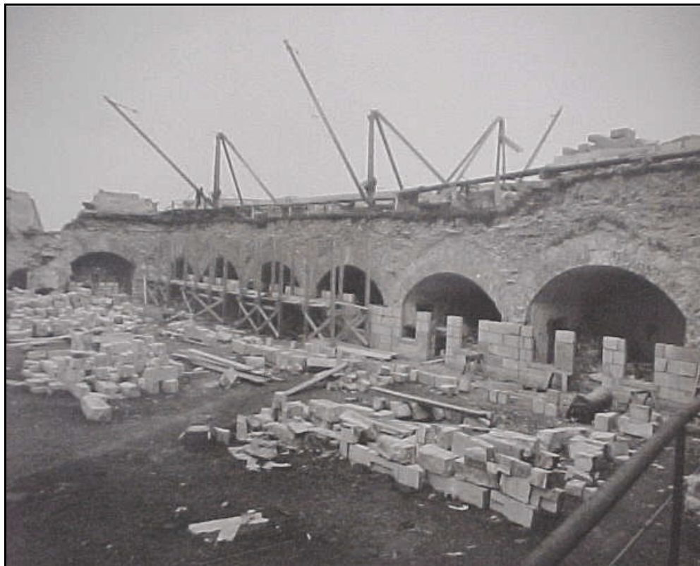
Figure 16 Rebuilding the wall west officers' casemates. Fort Henry Archives.
