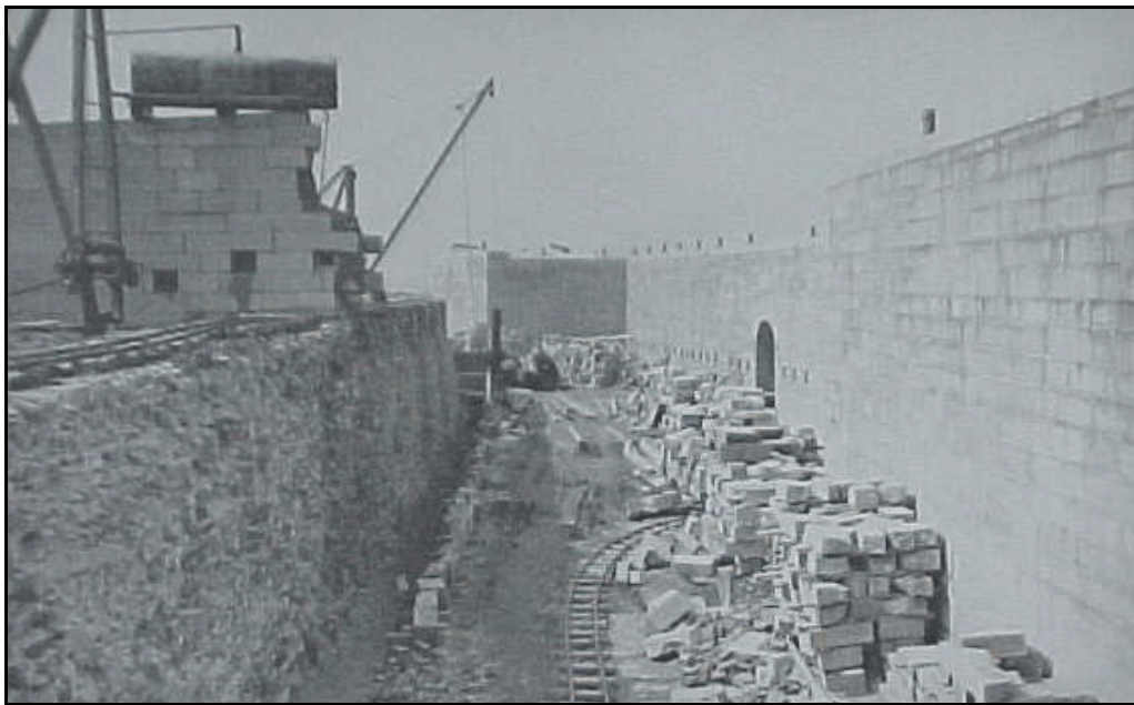
Figure 15 Reconstruction of south counterscarp wall; south curtain wall has been completed. Fort Henry Archives.
