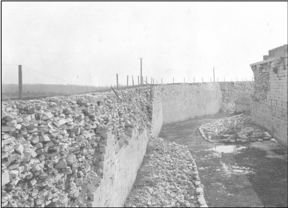
Figure 5 North ditch looking northeast, 1922. Parks Canada, 1205.
