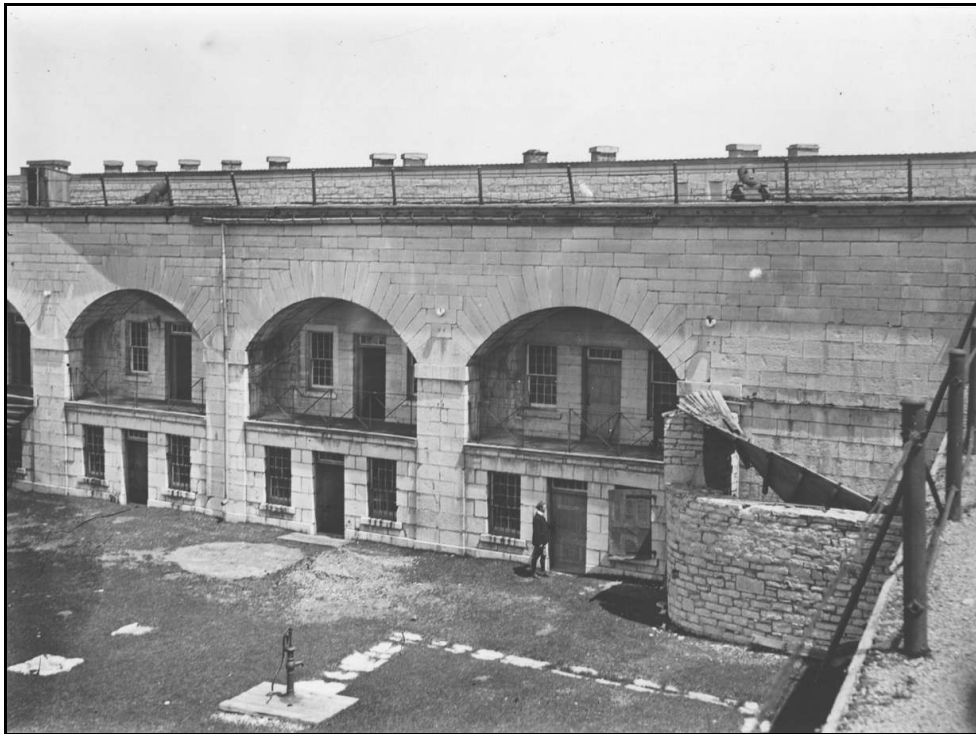
Figure 7 Northeast corner of the Redoubt, circa 1910. Note the powder magazine blast wall, with collapsed roof, and the pump into the water tanks. Marsden Kemp, Ontario Archives, 10003975.
