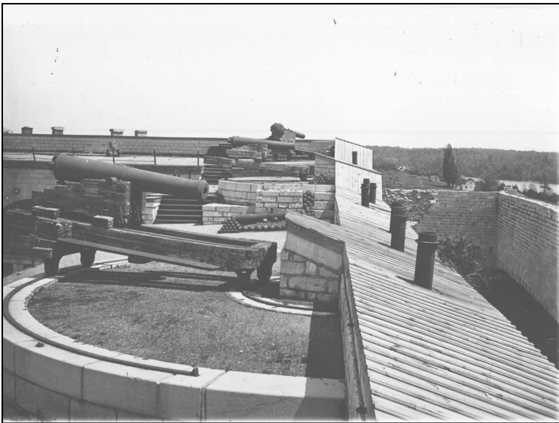
Figure 8 East ramparts of Fort Henry with 24-pr. gun on dwarf traversing platform in foreground, Armstrong gun to the rear, circa 1910. Note the board and batten covering of the parapet. Marsden Kemp, Ontario Archives, 10003974.
