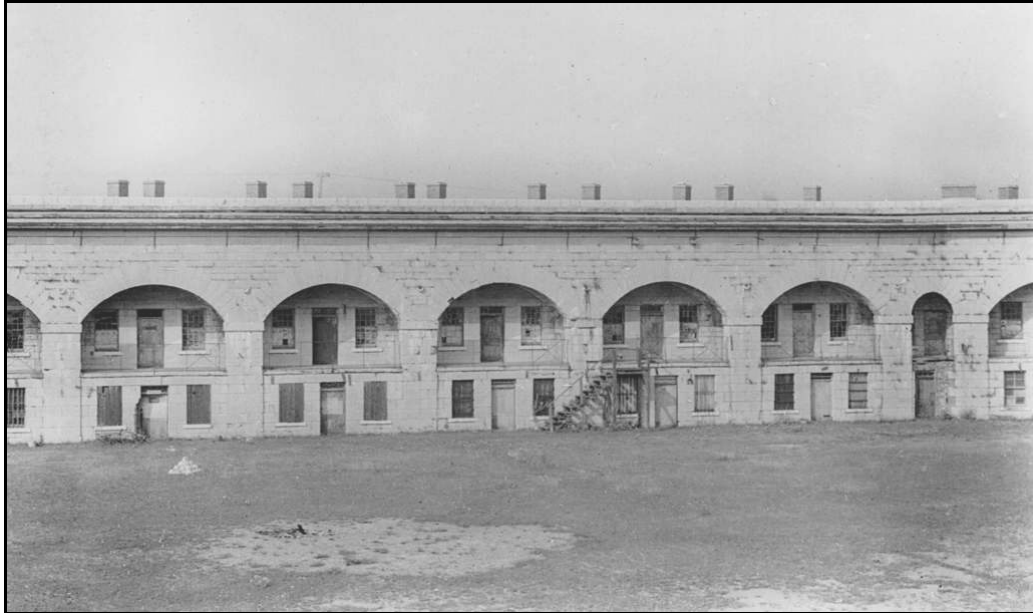
Figure 10 Part of north casemates; note roof. Stairway possibly left over from POW camp. Eric Arthur, Ontario Archives, C57-2-56_1.
