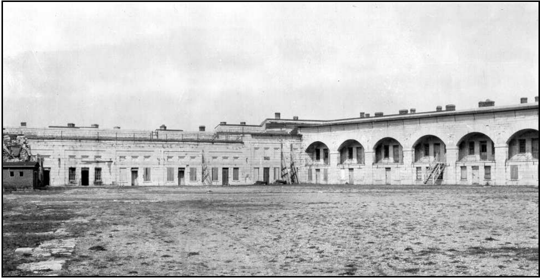
Figure 6 West and north casemates, 1922. Cf Figure 8. Parks Canada, 1206.
