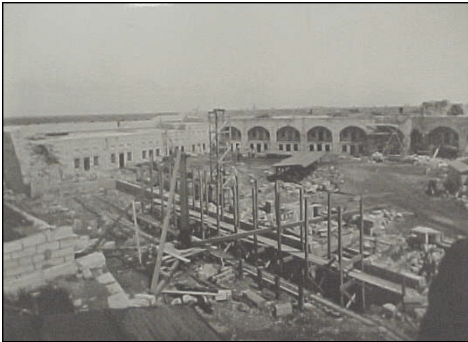
Figure 14 Beginning to build the south curtain wall. Facing on west casemates completely rebuilt. Some work being done on north casemates. Fort Henry Archives.
