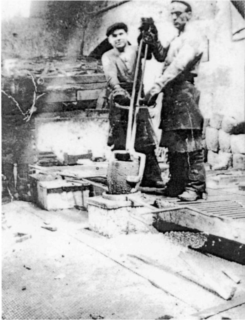
Workers at the brass foundry's crucible furnace in 1909. They used long-handled lifting tongs, and a two-men shank, a tool with which the crucible was carried to fill the moulds.
