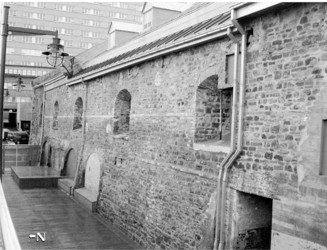
The east end of Chaussegros de Léry's curtain wall – the New Barracks' current north wall – where five of the original 17 cannon embrasures can still be seen. PHOTO: PARKS CANADA / R. GAUVIN.
