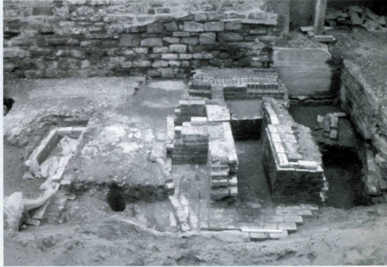
Western section of the reheat furnace constructed in 1902-1903. PHOTO: PARKS CANADA / A. NAULT.
