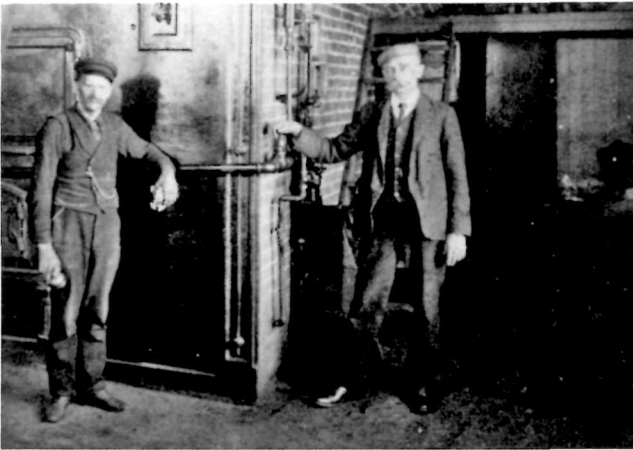
The room housing the boiler for the loading workshops on the Plains of Abraham 1902 Photo : Public Archives of Canada
