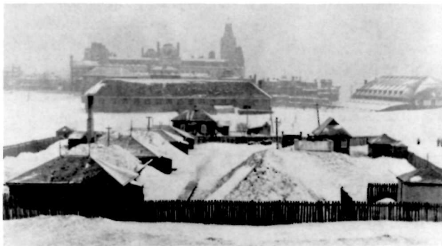
Overall view of one of the loading and assembly workshops on the Plains of Abraham (Cove Fields)
