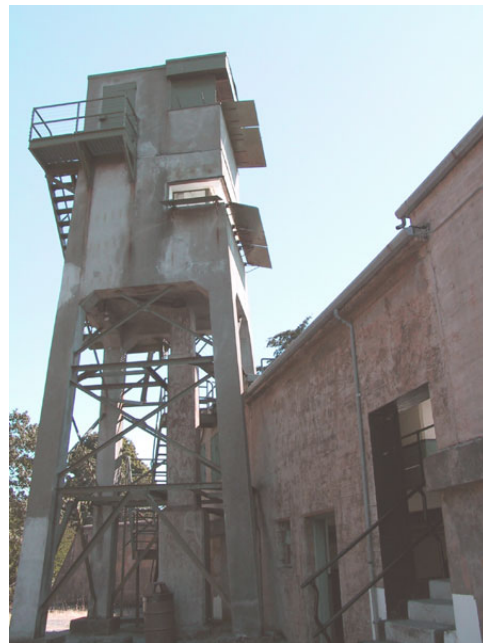
Belmont Battery - Director's Tower A. Gavin, WCSC 2003
