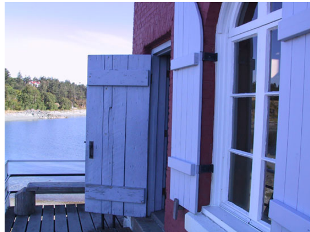
Fisgard Lighthouse A. Gavin 2003
