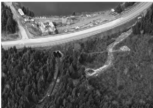
Bennett Lake Dam reconstruction. Chris Reardon
