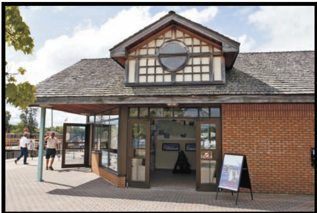
Parks Canada Welcome Centre, Port Severn
