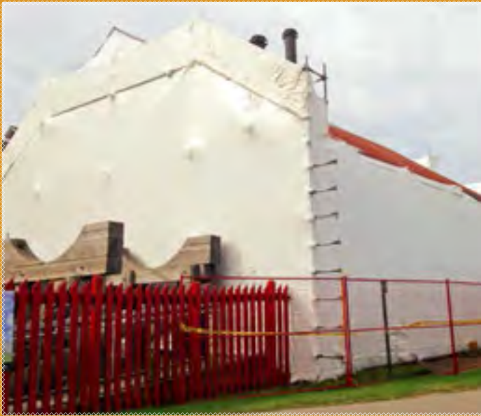
Above photo: Oil Drum Storage building during repairs.
