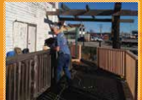
Photograph above: Construction of new harbour viewing deck
