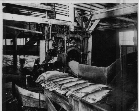
Figure **3B-Upper**Sliming tables for washing fish after they are butchered
