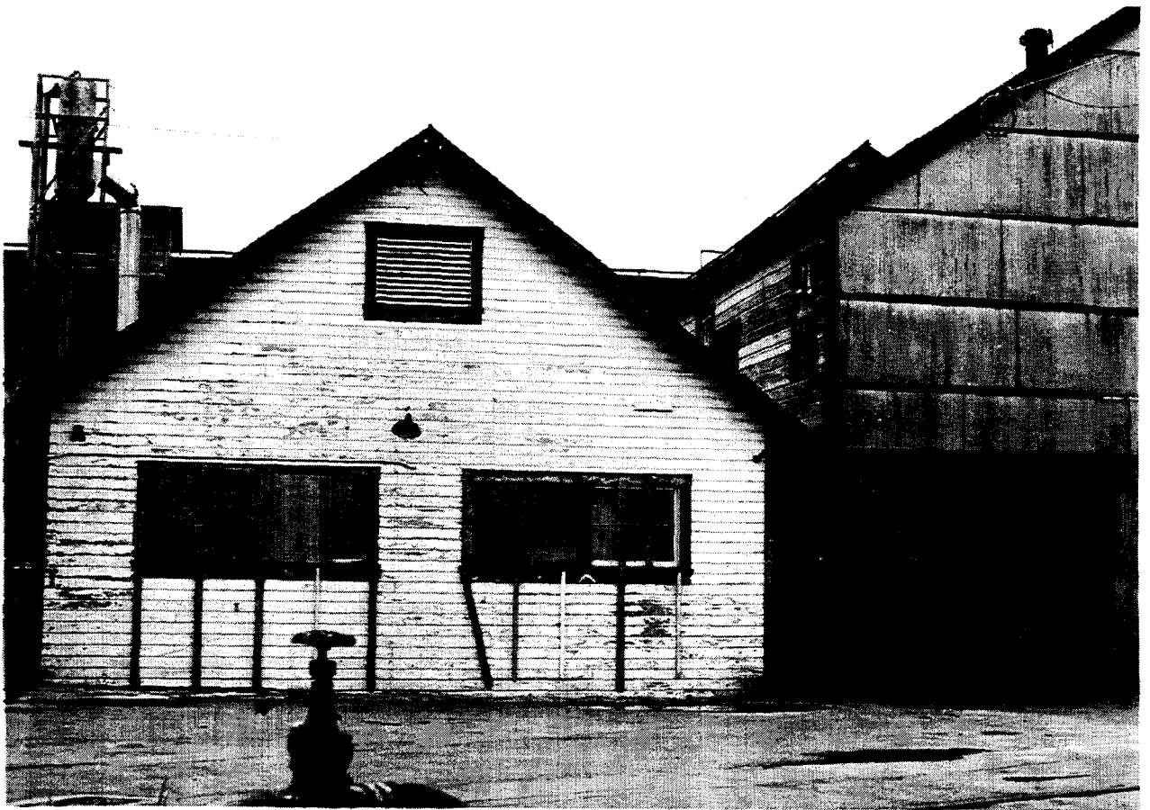
VITAMIN OIL PLANT EAST SIDE, NORTH ADDITION ON RIGHT AND MAIN SECTION OF ORIGINAL CANNERY IN BACKGROUND, 1982.
