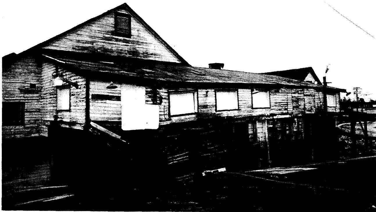
SOUTH SIDE OF MAIN CANNERY BUILDING, 1982. HERRING BINS WITH ORIGINAL (CIRCA 1906) SOUTH FACE IN BACK.
