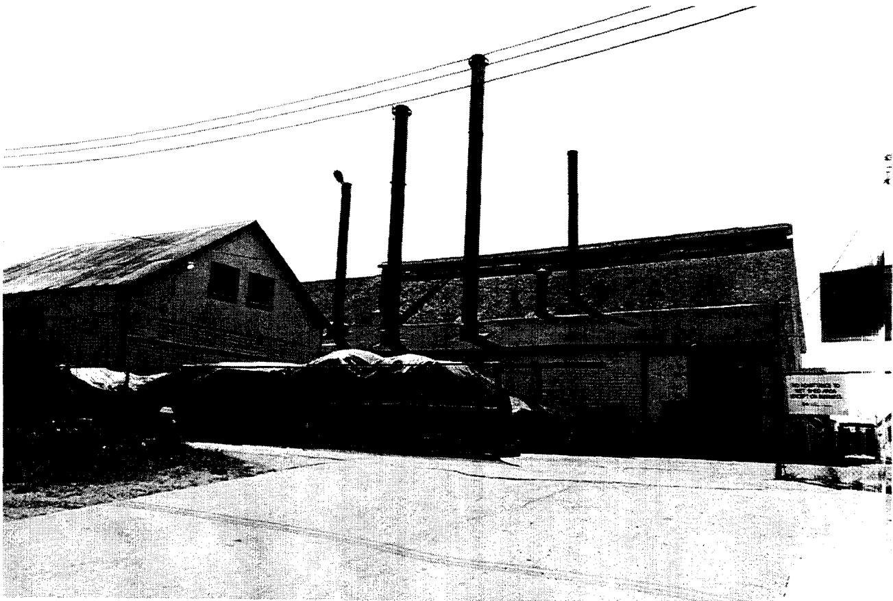
NORTHWEST CORNER OF MAIN CANNERY BUILDING, DRUM SHED ON LEFT, 1982.
