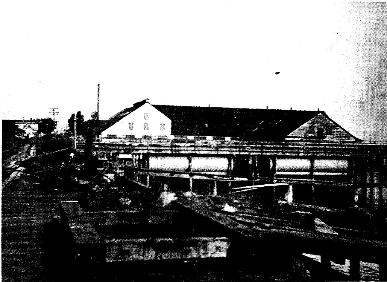
WEST SIDE OF THE MAIN CANNERY BUILDING, WEST WING ON RIGHT, 1926-30.
