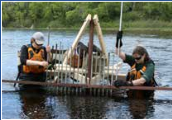
Resource Conservation staff constructing a fish fence.
