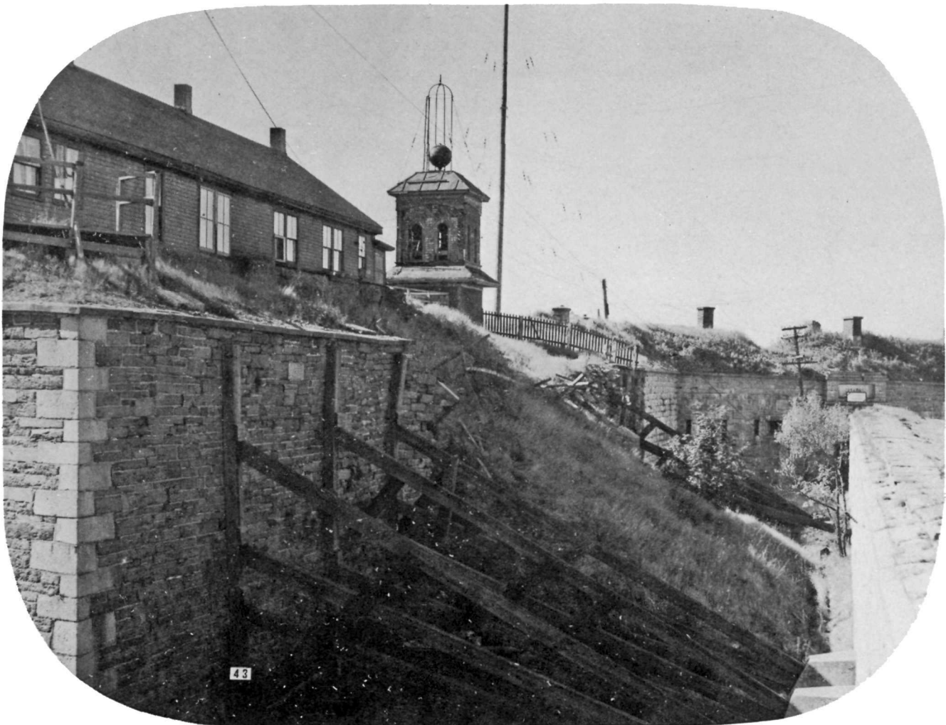
Deteriorated Wall in 1950 Public Archives of Canada
