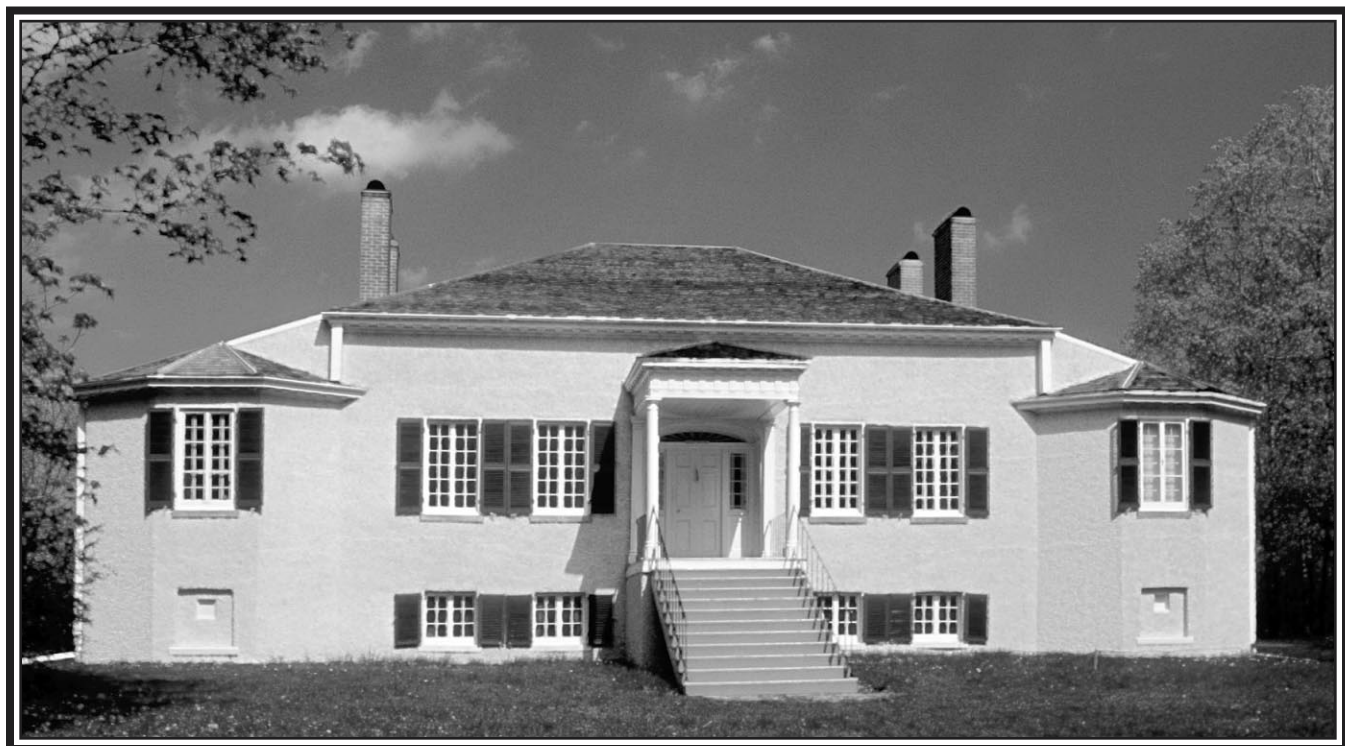
Facade of Inverarden House illustrating Regency design elements
