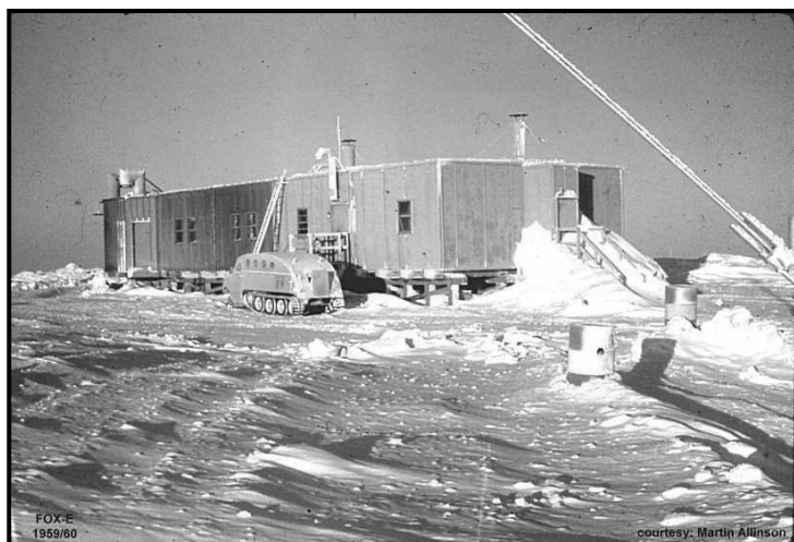
Module building at DEW Line site FOX-E (Durban Island/Padloping, NU) c1959/60. From DEWLiner website.
