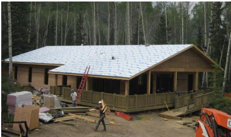
New accommodation building under construction at the Palisades Centre.
