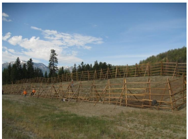
Erosion-control and re-vegetation work along the TMX pipeline right-of-way.
