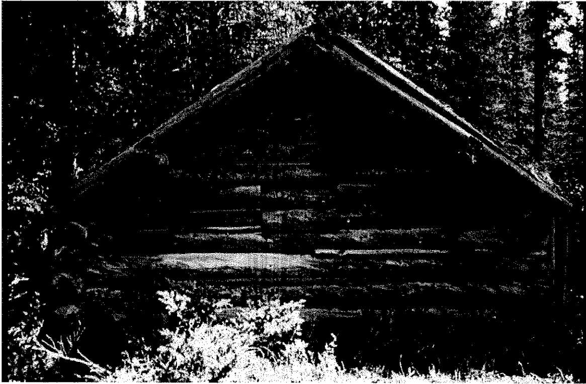
Figure 6. West-facing wall of the Glacier Trail Cabin. Increment core samples were collected from the three lowest logs shown.
