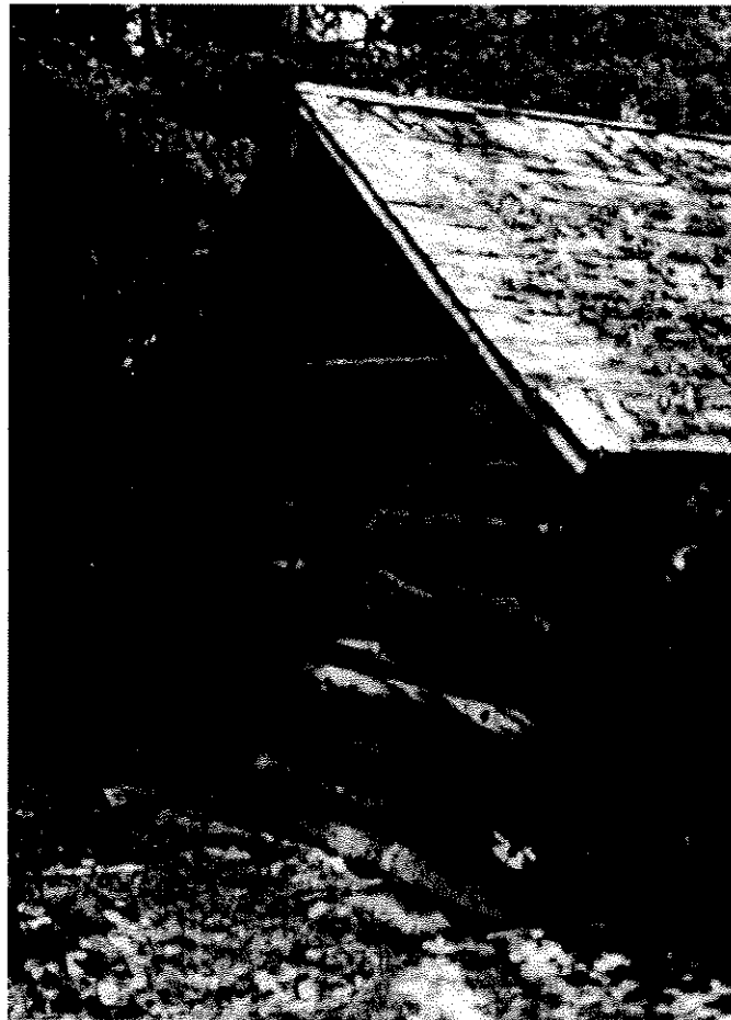
Figure 9. West-facing wall of the Hector 9 Mile Warden Cabin that overlooks Hector Lake. Exterior logs show evidence having been burned.
