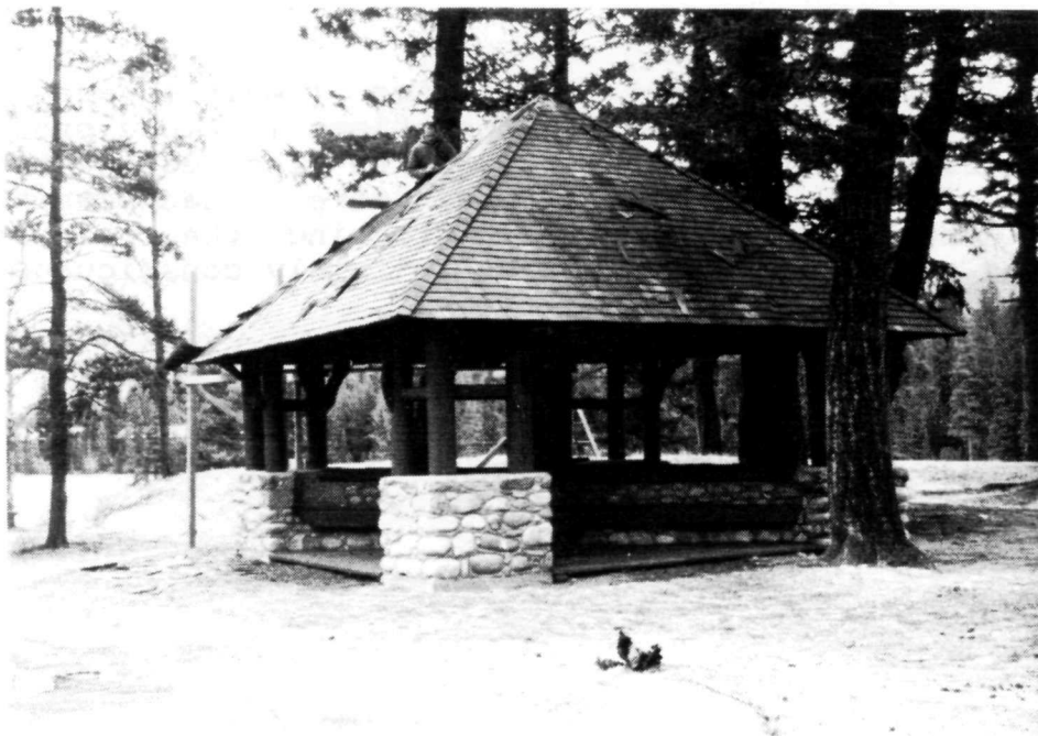
Figure 22. Log and stone golf shelter, with notable log truss system. (P. Buchik, 1992.)
