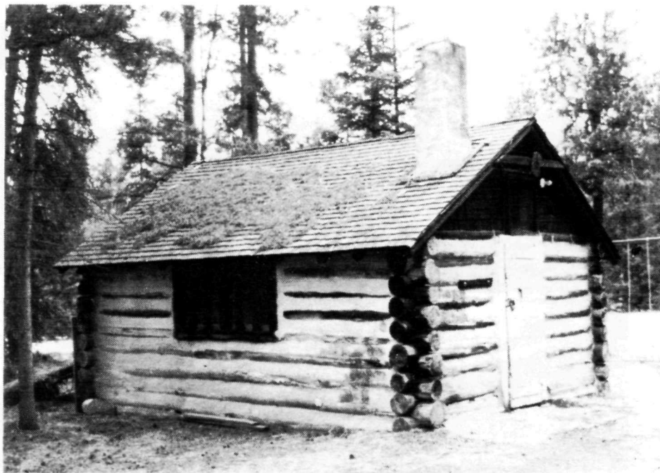
Figure 27. Log cabin, built ca. 1924 by Fred Brewster, presently part of Sky Line Trail Rides cluster. (P. Buchik, 1992. )
