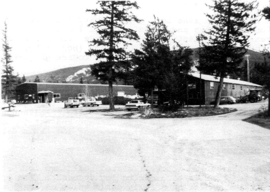
Figure 23. Metal-clad maintenance buildings, Zone H, erected in mid-1970s. ( P. Buchik, 1992. )
