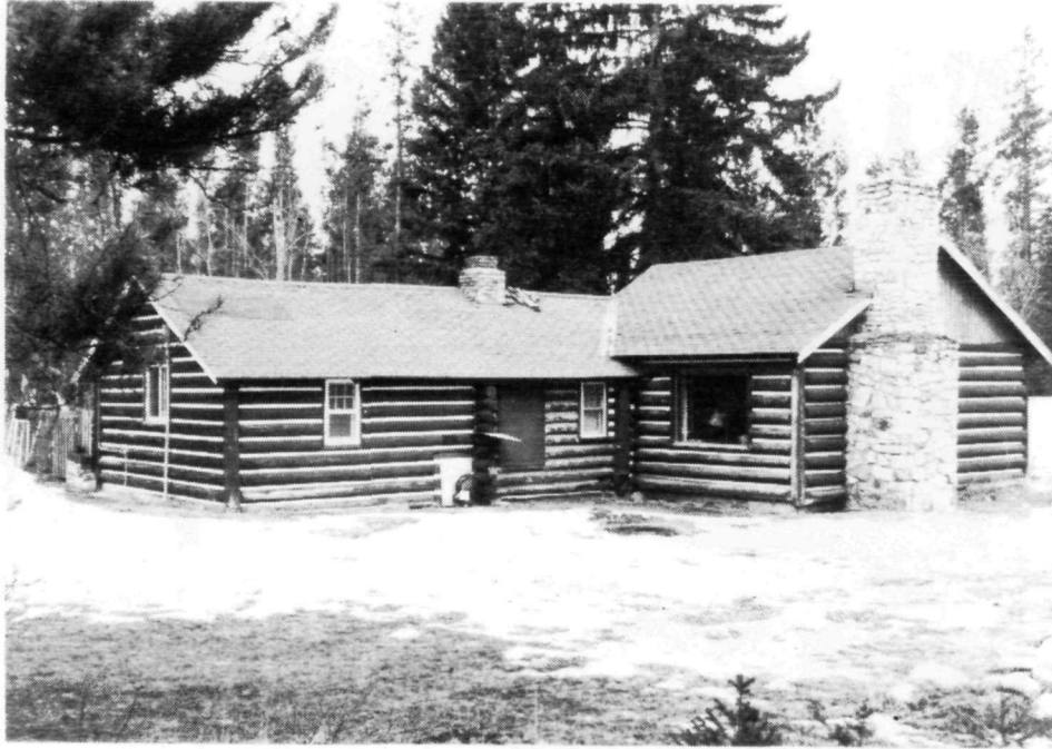
Figure 28. Building supervisor's residence, one half built in 1921 as part of Brewsters' Tent City resort. (P. Buchik, 1992.)
