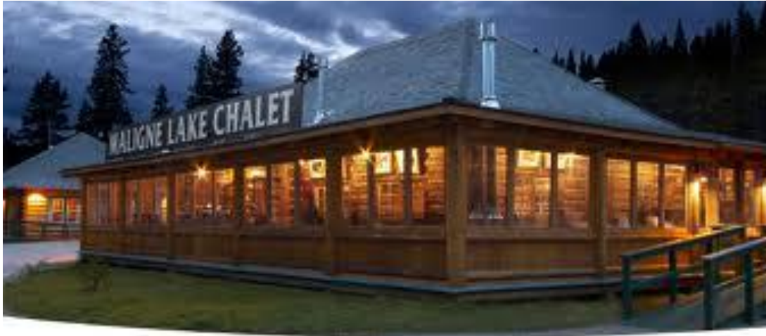
Figure 7 – MTL’s Restored Maligne Lake Chalet
