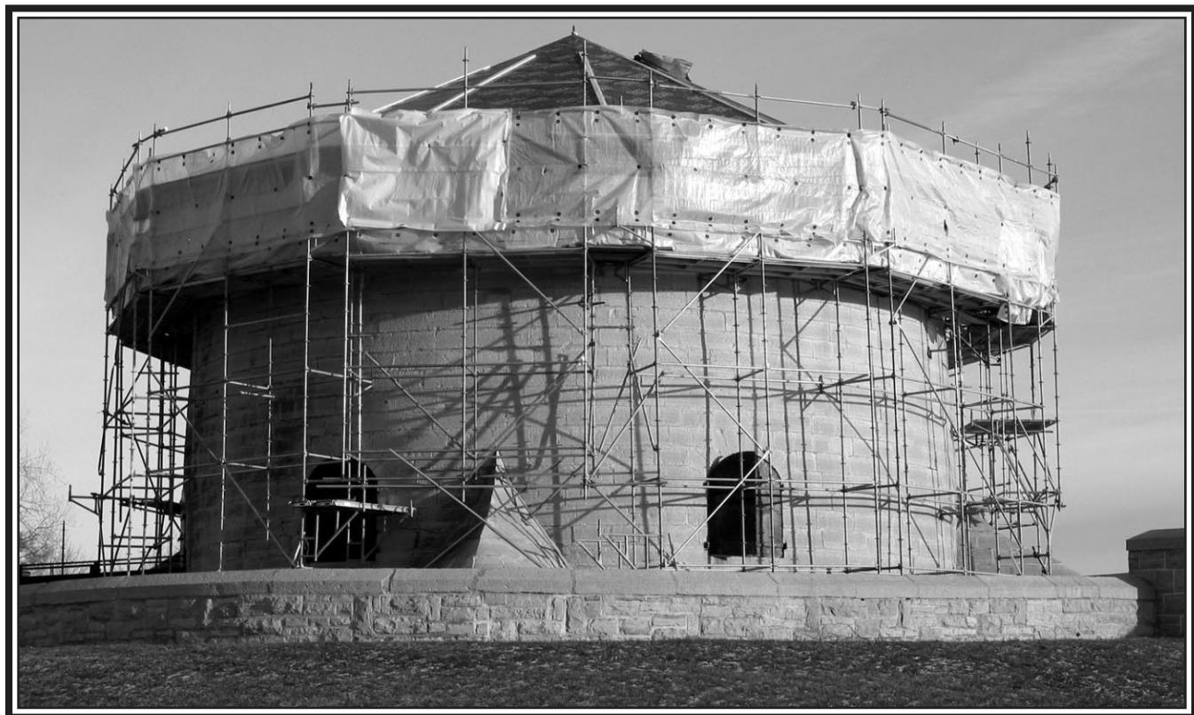
Roof restoration in 2003, Murney Tower, Parks Canada
