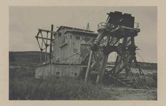
The first experiment with placer mining bucket elevator dredges was made in 1867 at Otago, New Zealand. This dredge was powered by current wheels. The first steam driven dredge for mining was constructed to operate on the Molyneux river, New Zealand in 1881.
