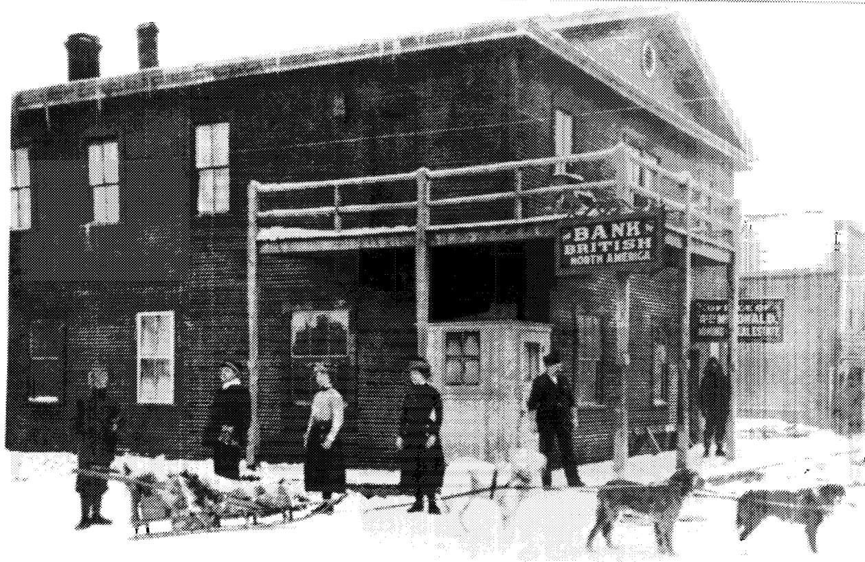
19 Bank of B.N.A., probably in winter of 1900-01; removeable winter porch is in place, but metal shutters have not yet been hung, and bottom portion of corrugated iron has not yet been painted in a darker shade of grey. (NA/AN - C53172.)
