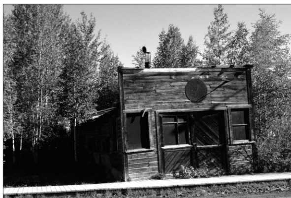
West's Boiler Shop
