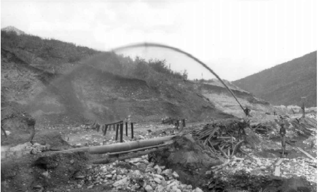
Hydraulic mining operations of the Pacific Coast Mining Co. on Cheechaco Hill - PC A Johns YT-223
