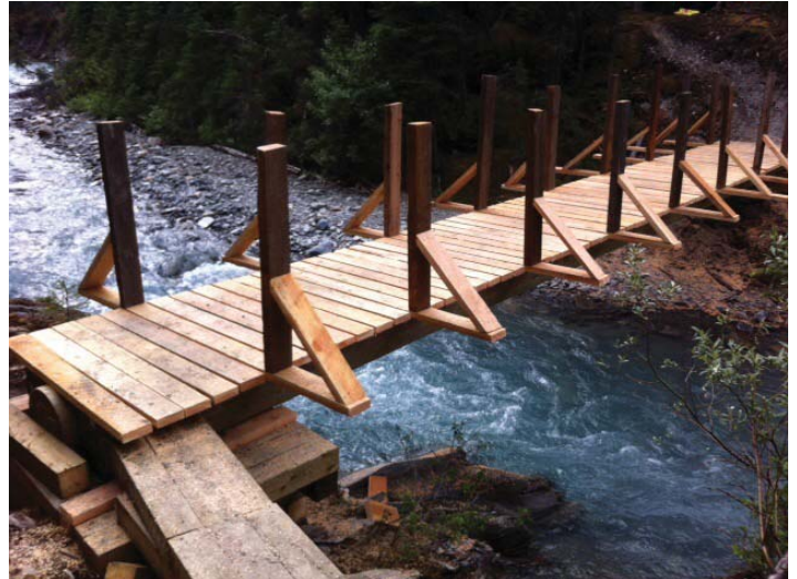
New bridge being installed over Numa Creek. (© Parks Canada / J. Hearnden)
