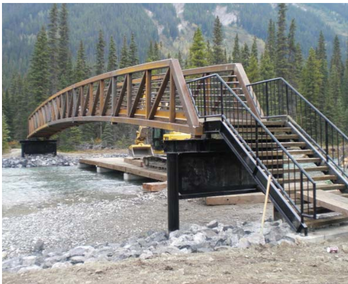
Paint Pots Bridge over the Vermilion River. (© Parks Canada / D McNamara)
