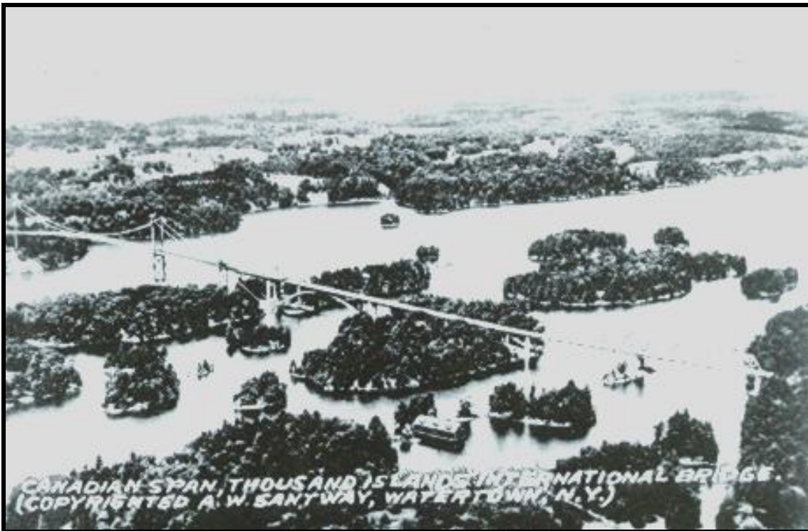
Figure 8 Canadian Span Thousand Islands International Bridge ca. 1935 NA, PA 194756
