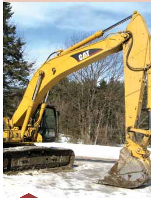
Heavy equipment on site for road building efforts in Gatineau Park. Photo: Michael Lait
