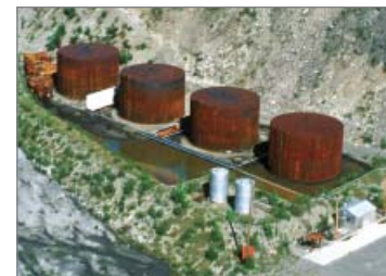
Fuel tanks at the proposed Prairie Creek Mine site
