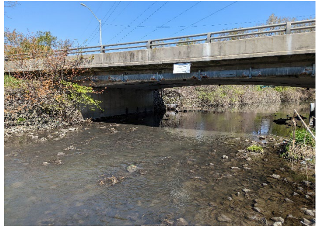
2. Todd Lane at the Turkey Creek bridge crossing.
