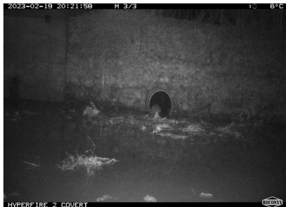
10. Raccoon entering small culvert on the west wall. February 19, 2023. (NE corner)
