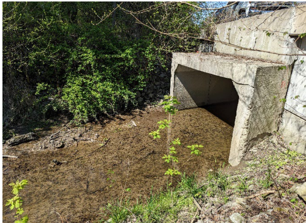
3. Basin Drain culvert under Malden Road (west).
