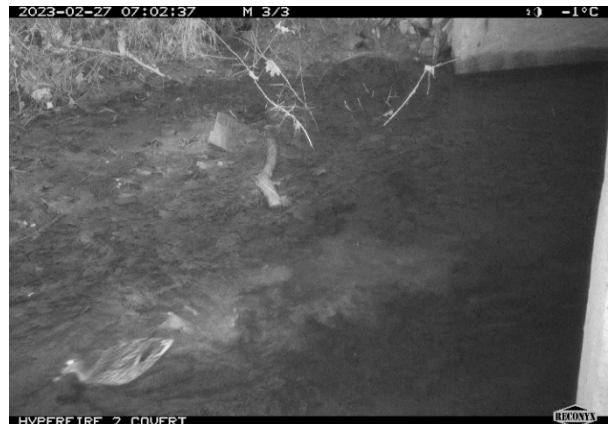
6. Female Mallards swimming out of the culvert west. February 27, 2023.
