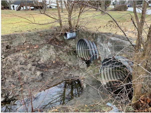
1. Basin Drain culverts under Spring Garden Road.
