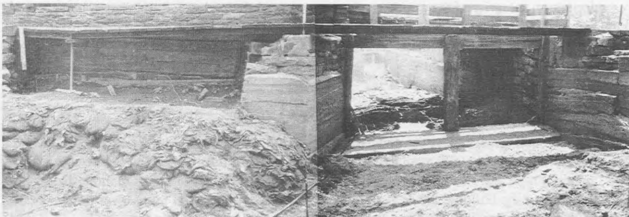
Fig.54 Northwest corner and dam frame during new dam construction (MNR Files)
