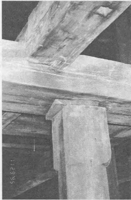
Fig.42 Relocated column detail
