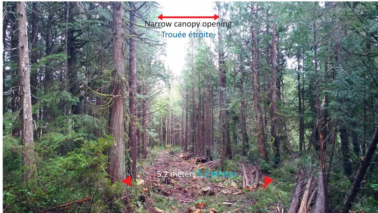
5.2 meter wide clearing to accommodate the trail. The clearing is wide enough to allow machinery to build the trail but narrow to limit impact of construction and overall footprint.
